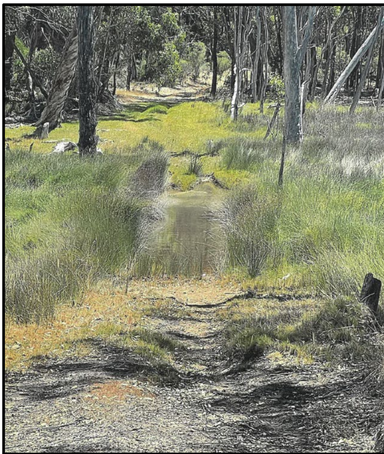
Above: Photograph of unconstructed (track) portion of Kenny Road
