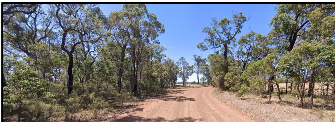
Above: Kenny Road turns into Poison Hill Road (at a bend). It physically appears as if it is one connected road to drivers/users.
