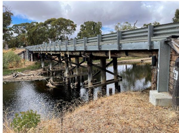
Figure 6 - LHS view of bridge 0274A
