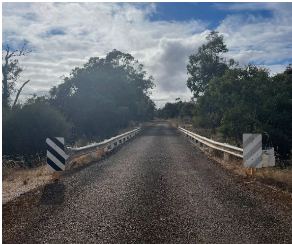
Figure 13 - Approach to bridge 4253A eastward facing
