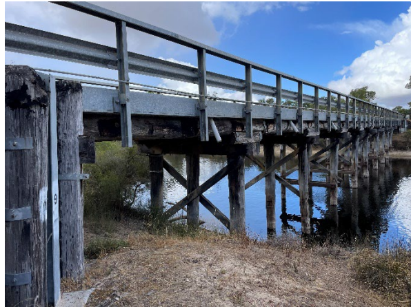
Figure 16 - RHS view of bridge 4254
