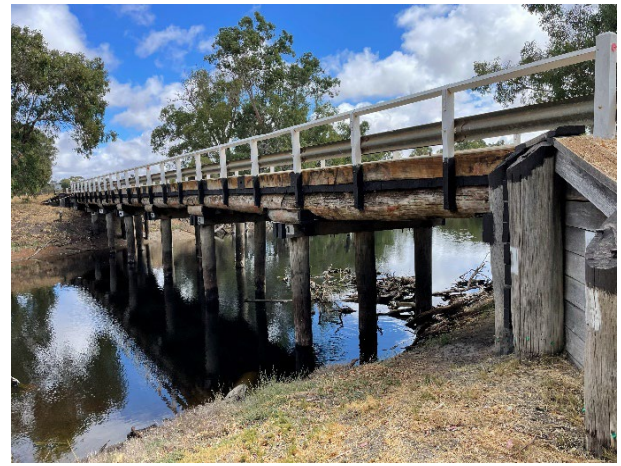
Figure 20 - LHS view of bridge 4256A
