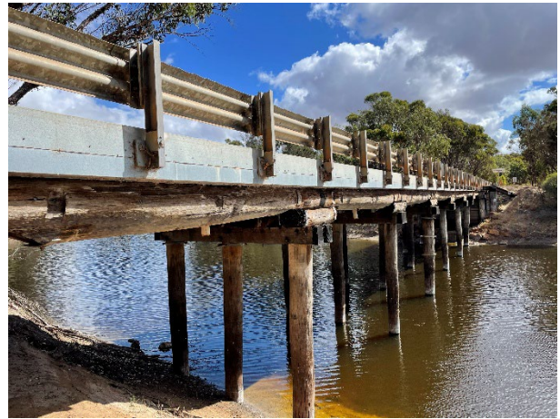
Figure 24 - RHS view of bridge 4258A.
