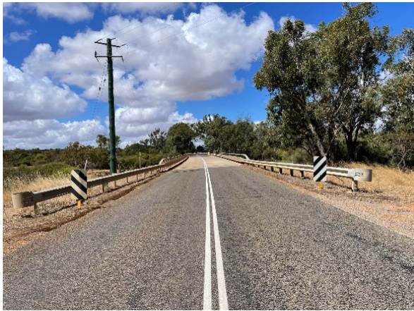
Figure 17 - Approach to bridge 4255A eastward facing
