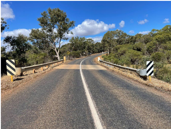
Figure 9 - Approach to bridge 0488 westward facing
