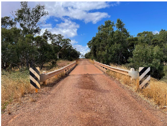
Figure 1 - Approach to bridge 0272 eastward facing
