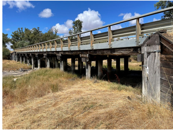
Figure 18 - LHS view of bridge 4255A
