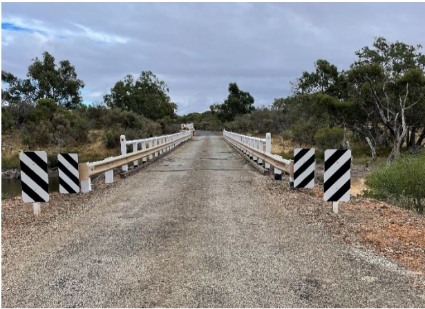
Figure 2 - Approach to bridge 0275A westward facing
