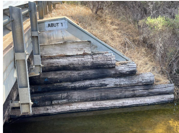
Figure 10 - Abutment 1 wingwall
