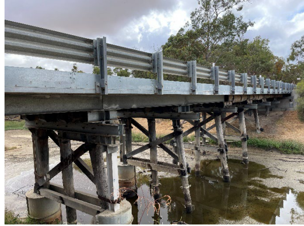
Figure 4 - RHS view of bridge 0273
