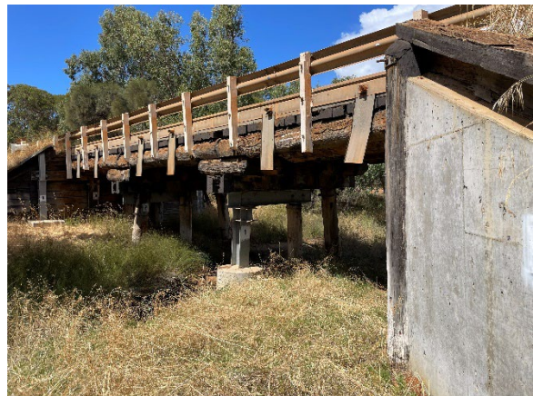
Figure 2 - LHS view of bridge 0272
