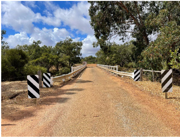
Figure 19 - Approach to bridge 4256A eastward facing
