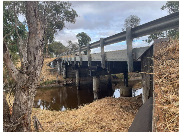
Figure 22 - LHS view of bridge 4257
