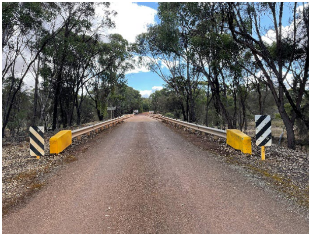
Figure 23 - Approach to bridge 4258A westward facing
