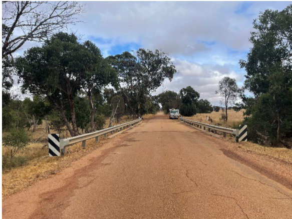
Figure 21 - Approach to bridge 4257 eastward facing
