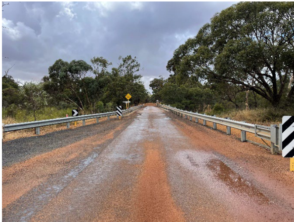
Figure 3 - Approach to bridge 0273 eastward facing
