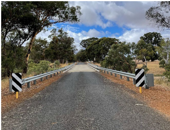
Figure 5 - Approach to bridge 0274A eastward facing
