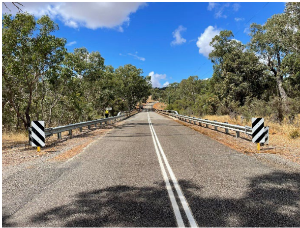
Figure 11 - Approach to bridge 0489 southward facing
