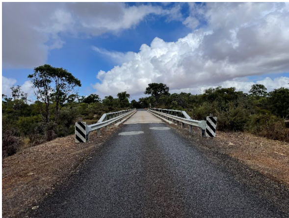
Figure 15 - Approach to bridge 4254 southward facing
