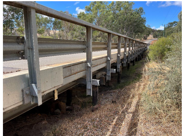
Figure 12 - RHS view of bridge 0489
