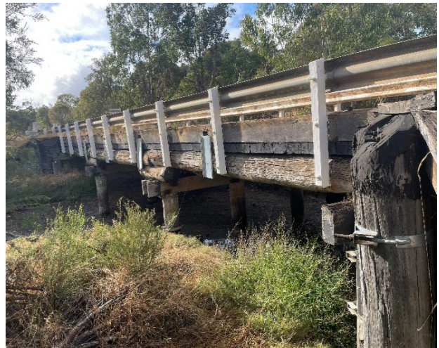
Figure 14 - LHS view of bridge 4253A
