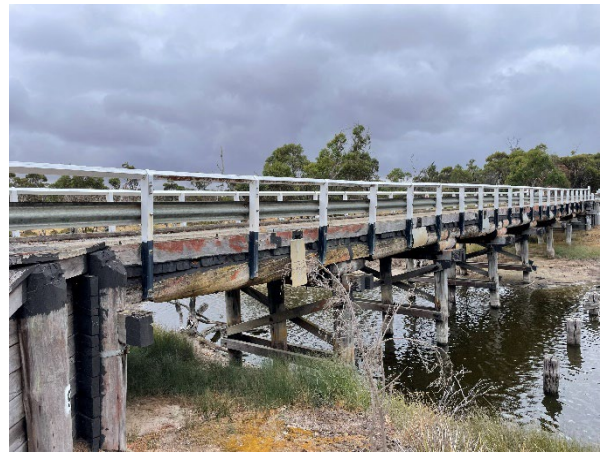
Figure 1 - RHS view of bridge 0275A
