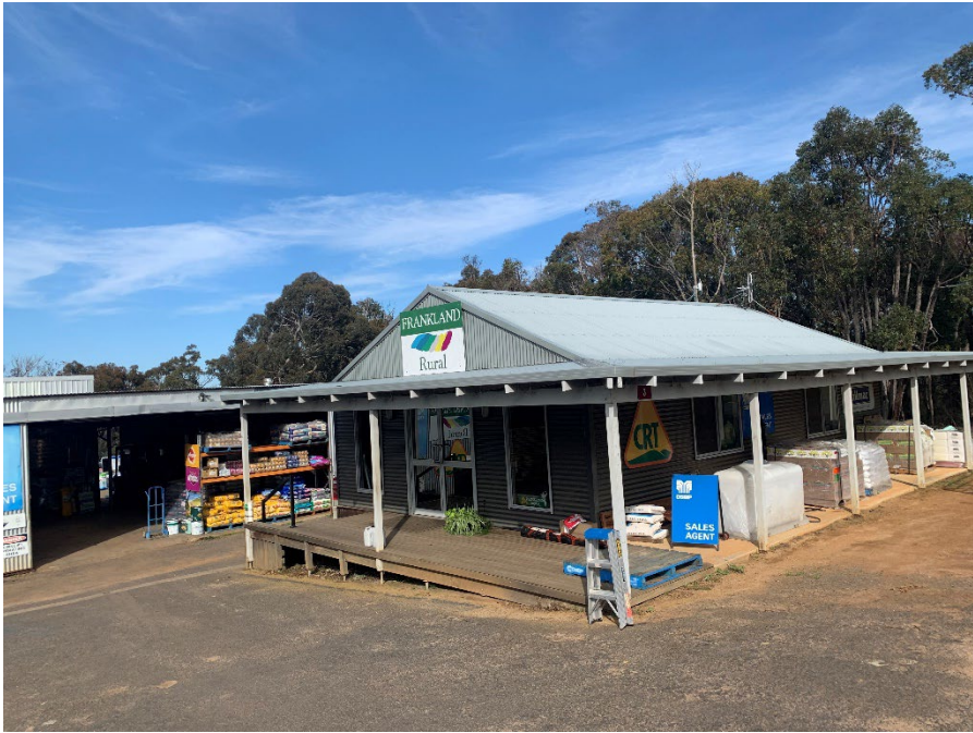
South Eastern Elevation of the existing Frankland Rural Office Building
